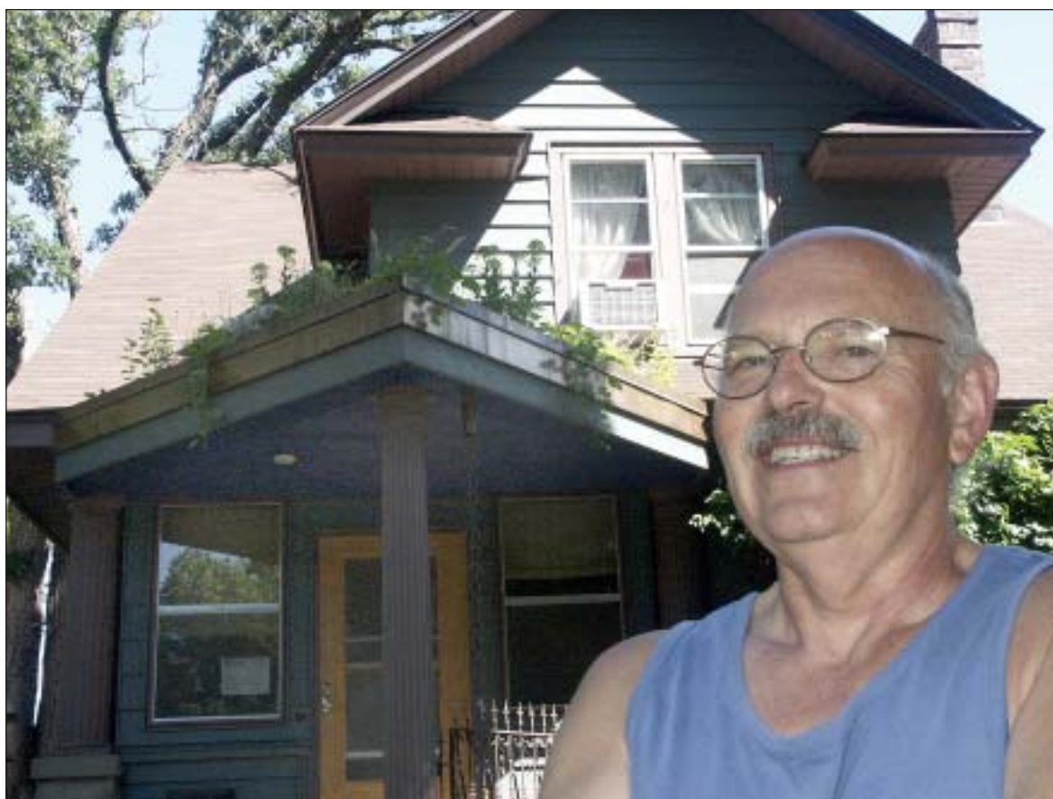
Last fall Hamline-Midway resident Terry Kormann, together with his wife Karen (not pictured), built a triangle-shaped roof addition on their three-season porch. Then they hauled 3/4 cubic yards of dirt up a ladder, spread it on the roof and planted a garden. (Photo by Terry Faust)
